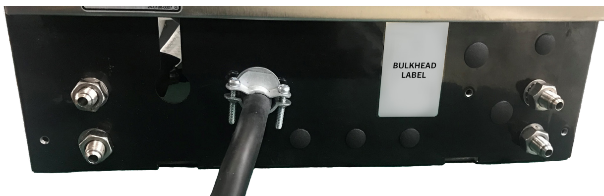
Figure 4.1 Bulkhead Fittings Label Location
